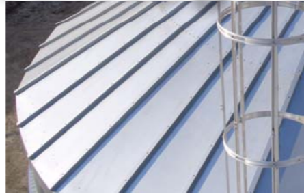
Silo roof without finish
