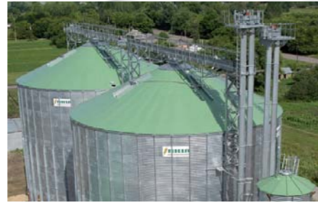
Silo roof with powder coating
